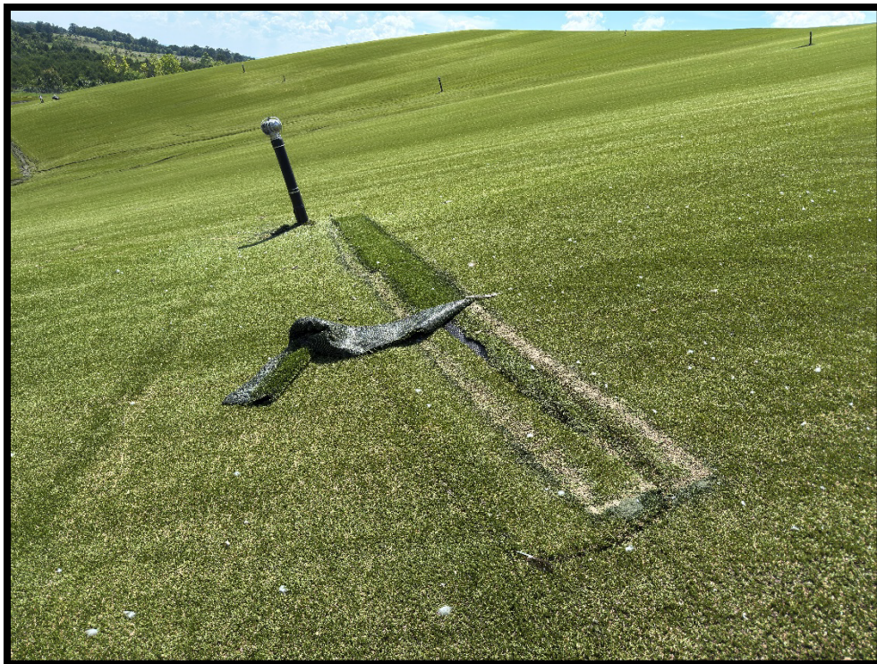
Photograph 4: View of damaged closure turf on the north side of Area 1-2.
